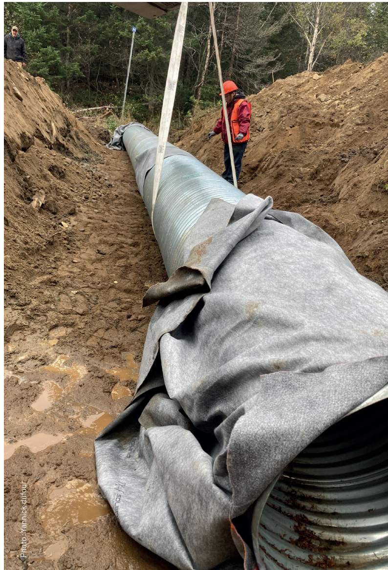
Installation de ponceaux
